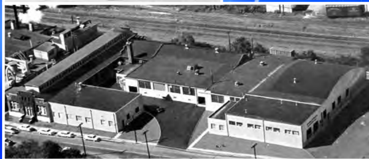
Boonton plant, New Jersey, 1950s-1960s.
