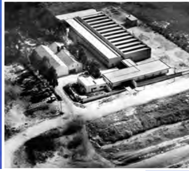
Construction of the São Paulo plant in Brazil, 1957.
