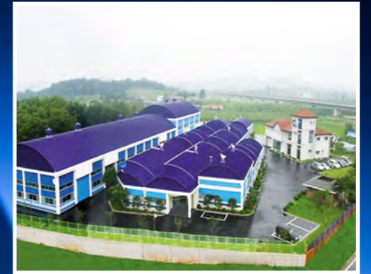
Inauguration of the Sangam plant in South Korea, 1991.
