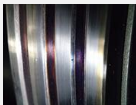
P42 – Oxidation of the metal
