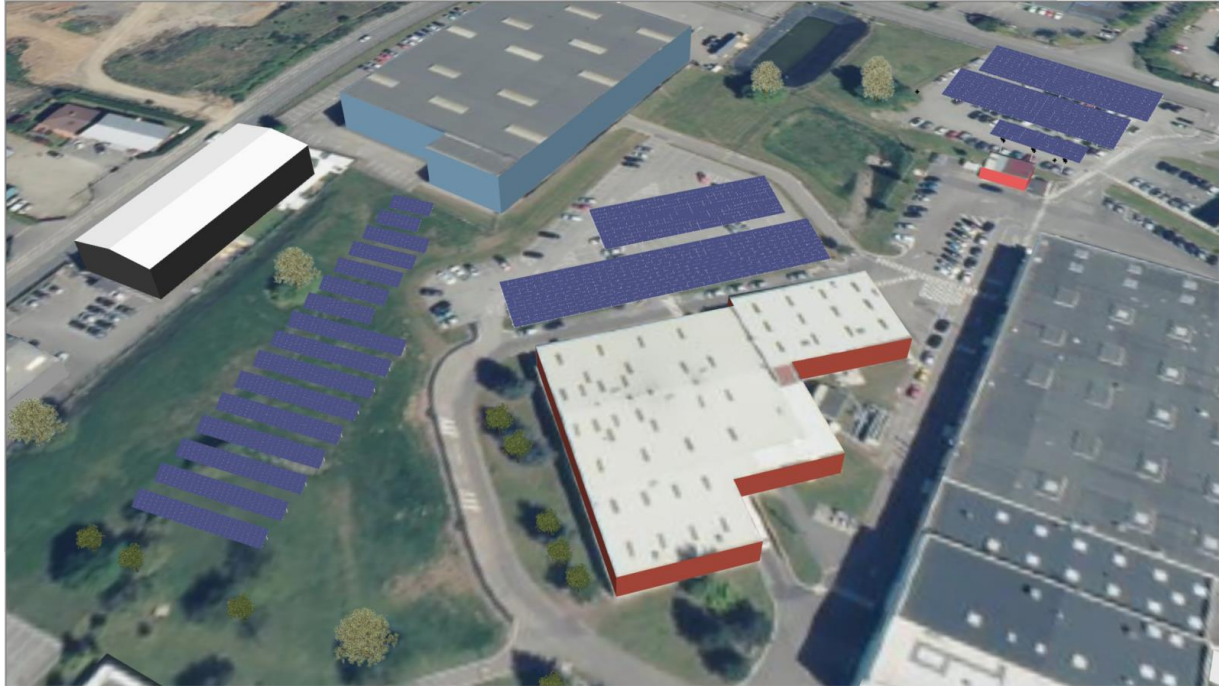
Location of the solar power projects – Mersen – Saint-Bonnet-de-Mure (France). Photo credit: Legendre Énergie
